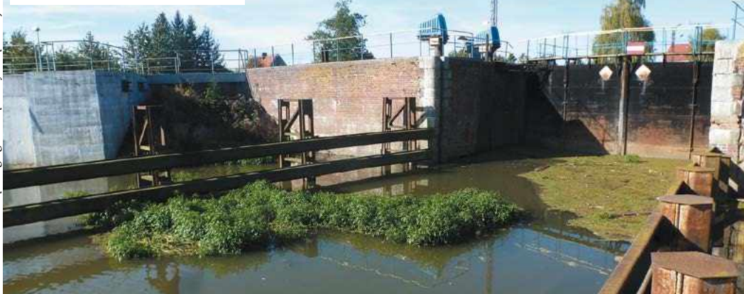
Closed left chamber of the Zwanowice lock
