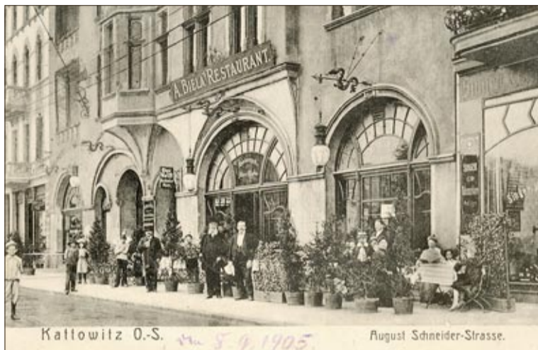
Biela's Restaurant 1905 Aussenansicht
