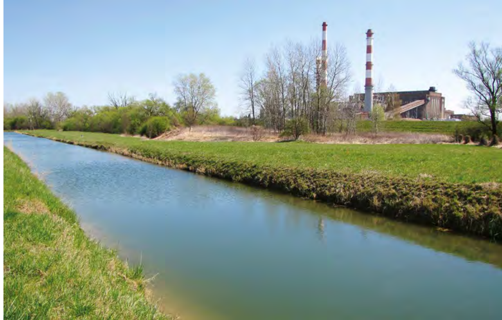
Additional groundwater supply from the Dunajec River through a infiltration trench in Tarnów / photo: Grzegorz Wojtal
